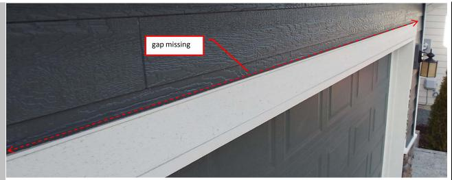
The new door at the West side of the home is not properly flashed at the top of the head jamb. I recommend evaluation/repairs by a qualified party.
