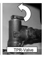
Typically a maximum of 4, 90 degree bends are allowed in the drain of the TPRV of the water heater--per valve manufacturer and water heater manufacturer recommendations. There are currently at least 6. Unless a way of terminating the drain to the exterior can be achieved with four or less elbows I recommend that it be properly terminated elsewhere. I recommend evaluation/repairs by a licensed plumber and/or bring to the attention of the builder/seller for proper repairs.
